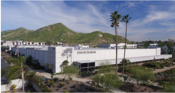
Bourns, Inc. Riverside, California U.S. Headquarters
