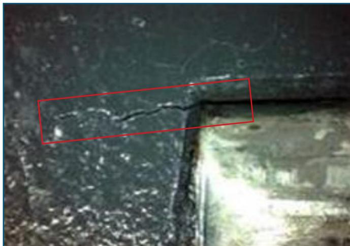
Figure 9 | *Acceptable Crack*
