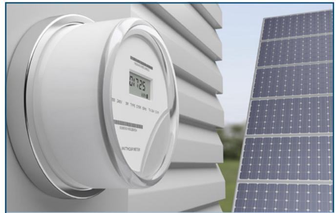
Figure 1. | Smart energy meters are typically found on the exterior of buildings and located on the AC mains line
